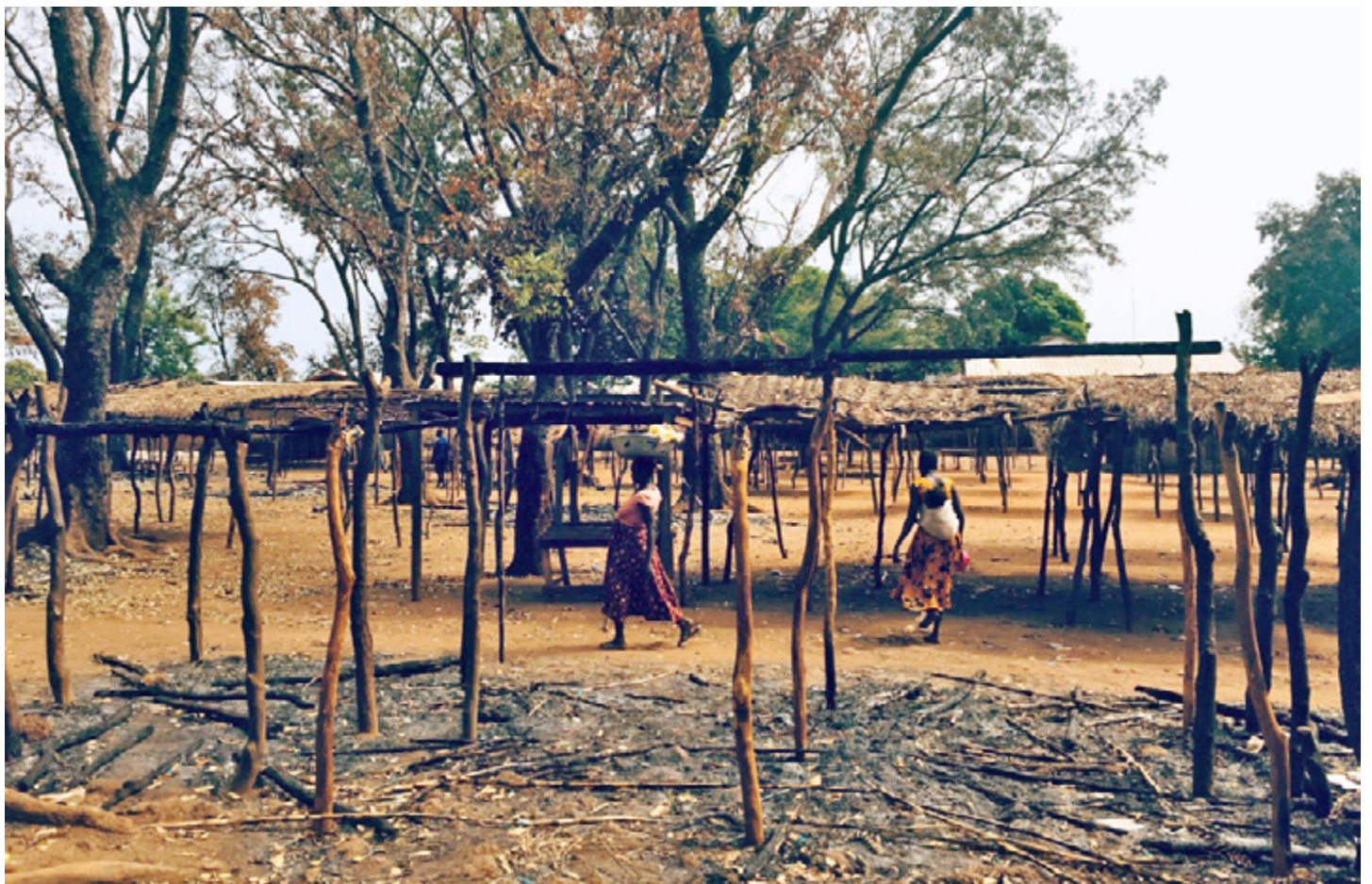
PICTURE 4. Burnt central market, November 1 st 2018.
